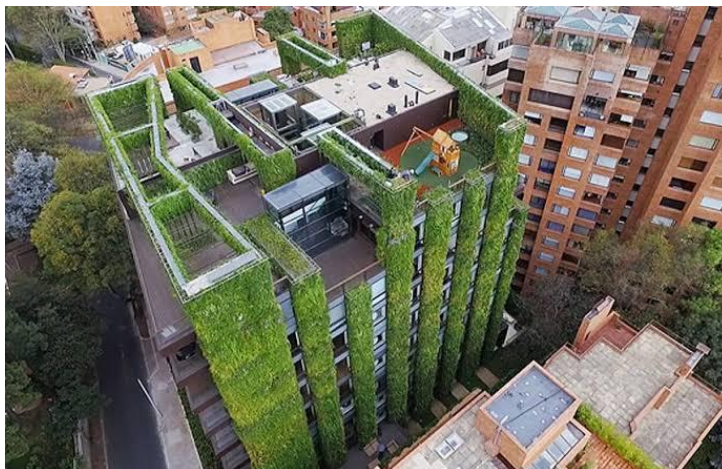
Figure 9 Bogota, Colombia_ World's largest vertical garden on multistorey residential building (115,000 plants) treehugger.com.
