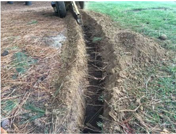
Figure 6 Tree root damage from service installation
