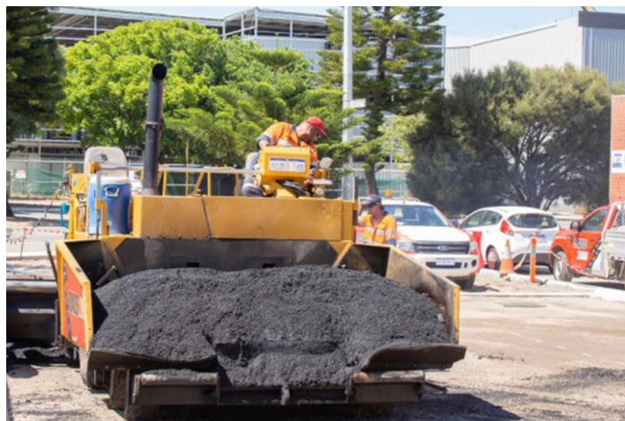
Figure 6: City of Fremantle carpark
